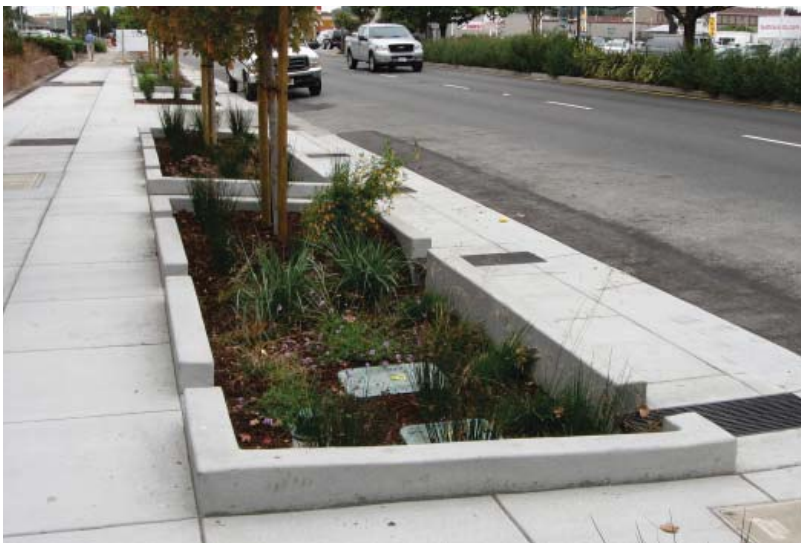
Bioswale with curb cuts to collect runoff, El Cerrito, CA
