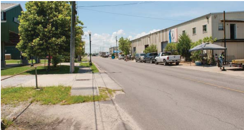
New sidewalks in front of Aycock Barn, at left, do not continue, while large curb cuts for off street parking, at right, impede pedestrian and bicycle access
