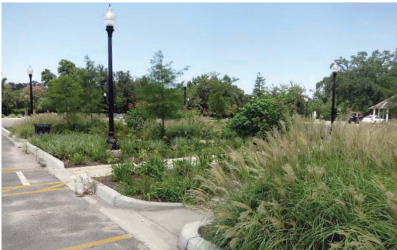
Bioswales and rain gardens clean parking lot runoff at City Park in New Orleans
