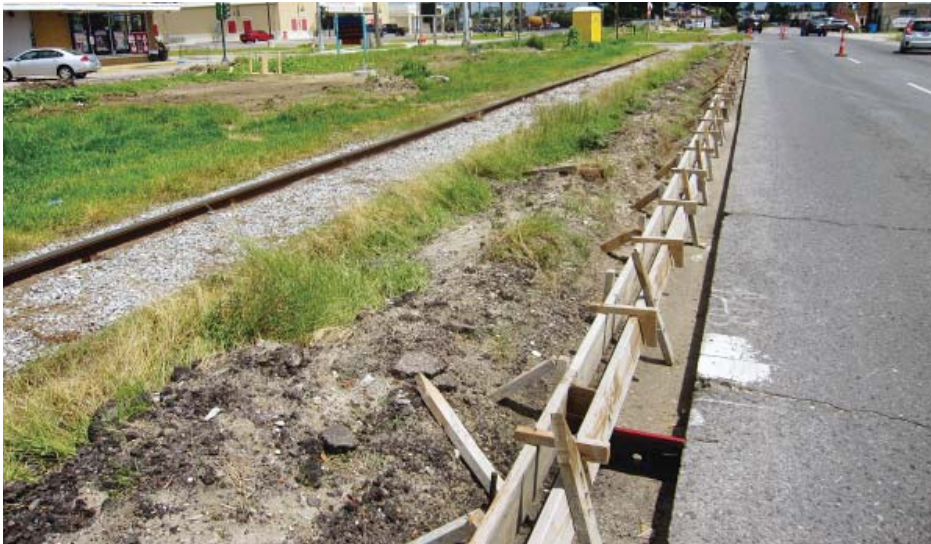
Formwork for new curbs, August 2016
