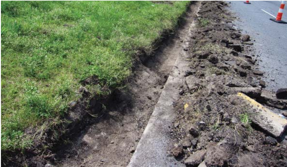
Demolition of curbs on St. Claude Avenue during construction of streetscape improvement project, August 2016
